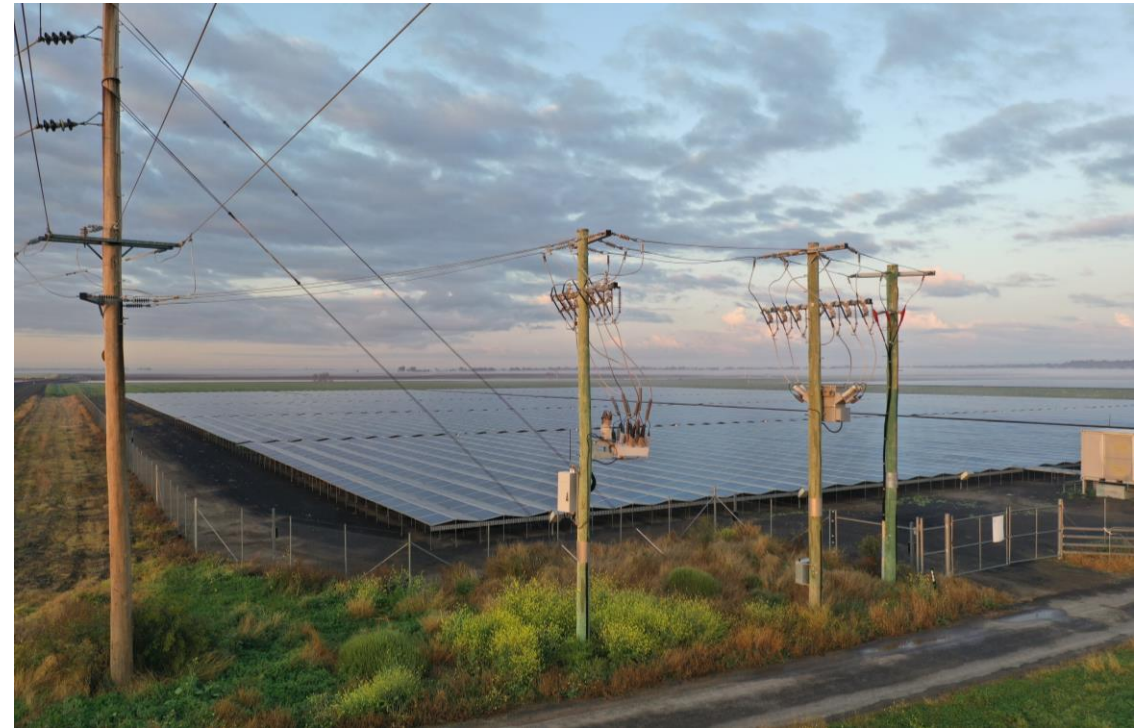
Goondiwindi Solar Farm – Overhead Connection with separate metering installation
