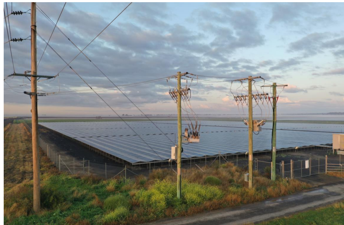
Goondiwindi Solar Farm – Overhead Connection with separate metering installation
