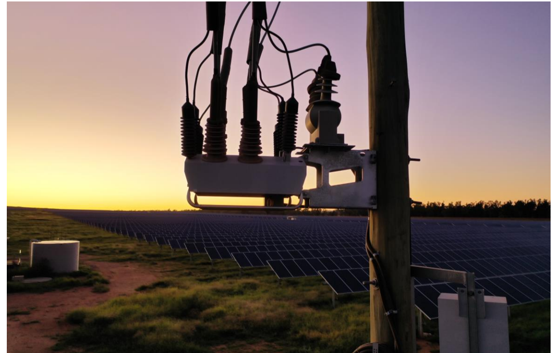
OSM Recloser Installation – Narrabri Solar New South Wales, Australia
