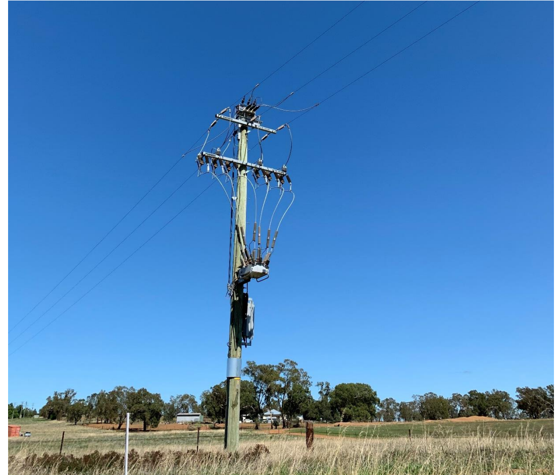
Recloser installation, NSW Australia
