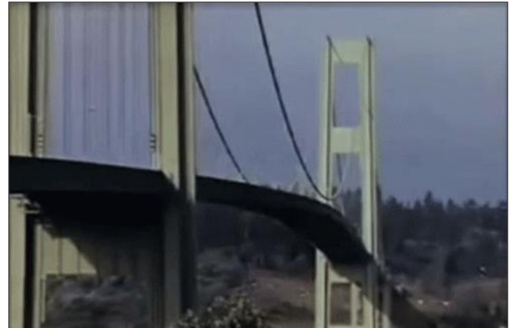
The Tacoma Narrows Bridge collapsed in 1940 due to poorly damped oscillations
