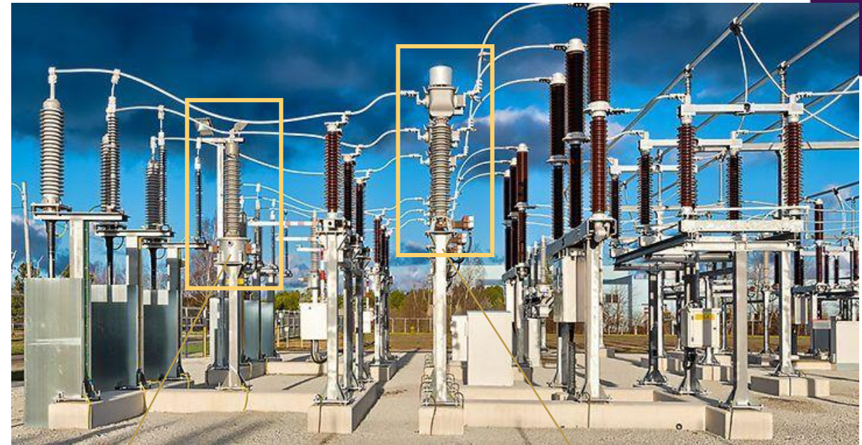
Voltage Transformer (input only)
